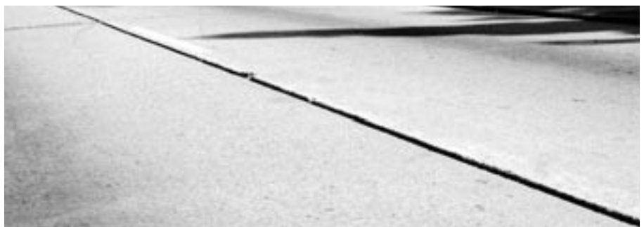
▲ Faulted longitudinal joint.
