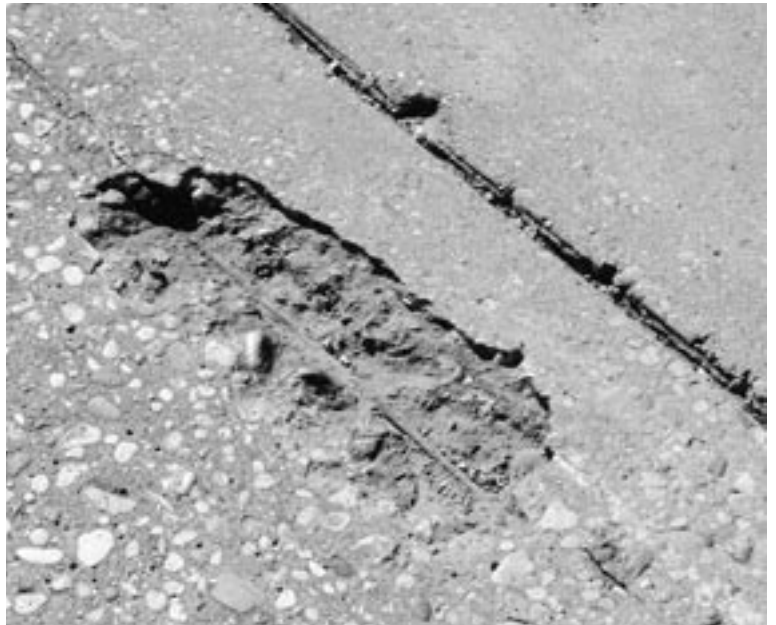
▶ Spalling over shallow reinforcing.
