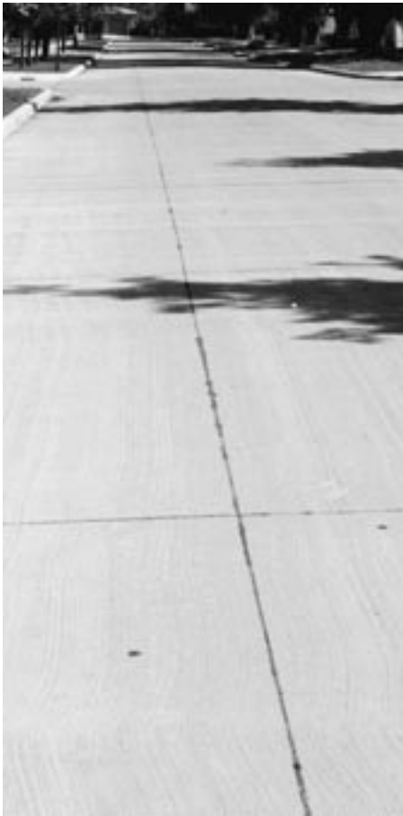
◀ New, well-sealed longitudinal joint.
