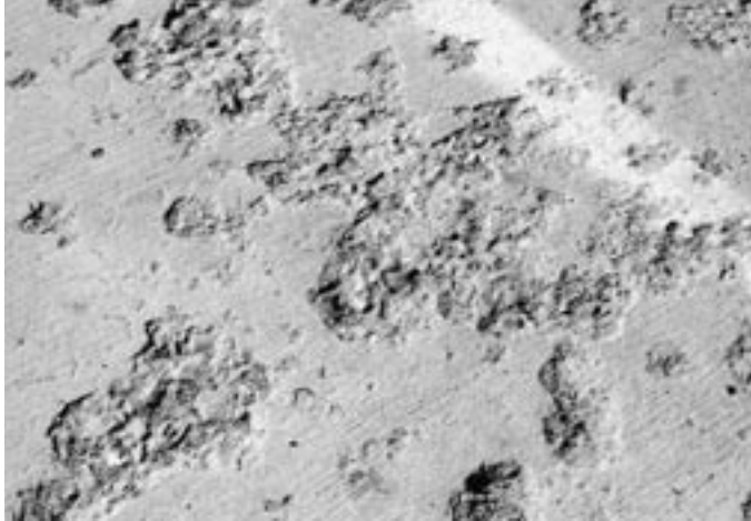
► Moderate surface scaling. Loss of mortar and fines from the surface beginning to expose larger aggregate.
