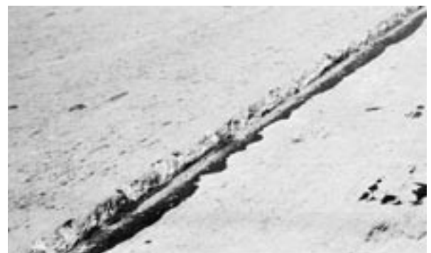
▲ Faulted longitudinal joint.
