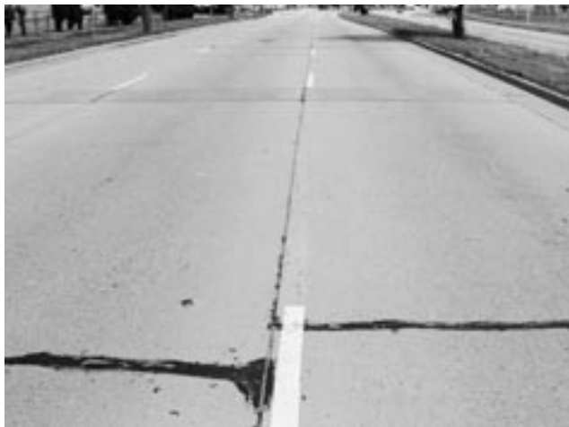
◀ Transverse crack. Tight, sound pavement.
