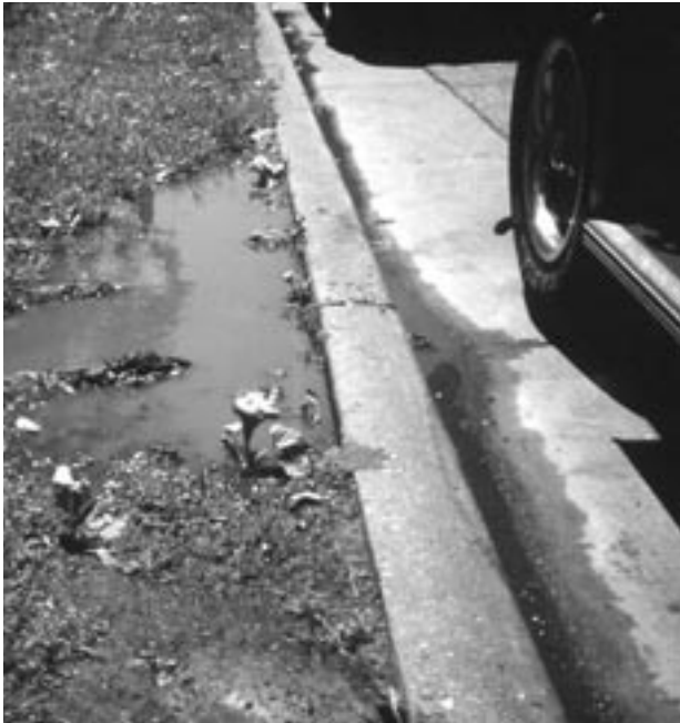
▲ Reshape terrace behind curb to restore drainage and prevent damage to curb and street.
