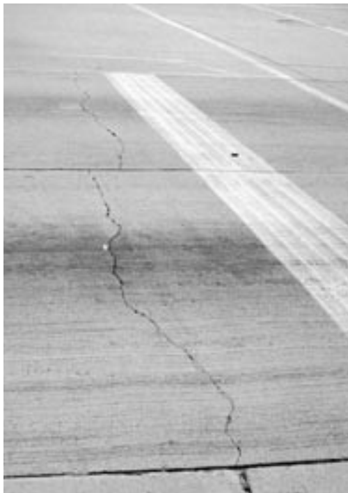
◀ Transverse crack. Tight, sound pavement.
