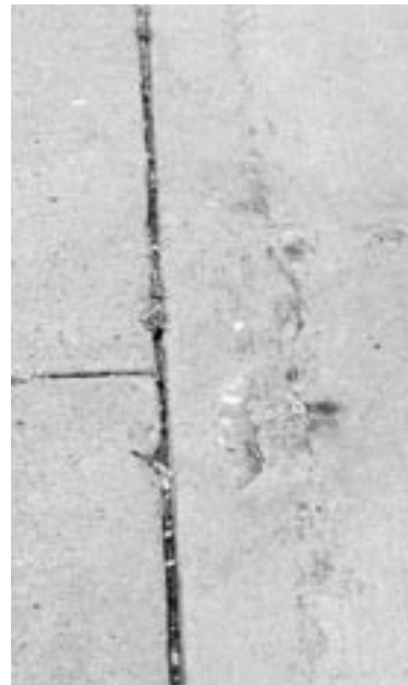
◀ Wire reinforcing mesh placed close to surface. Corrosion of the reinforcing steel causes the surface mortar to spall. Very difficult to patch and repair.
