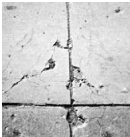
Corner cracking with broken concrete pieces.
