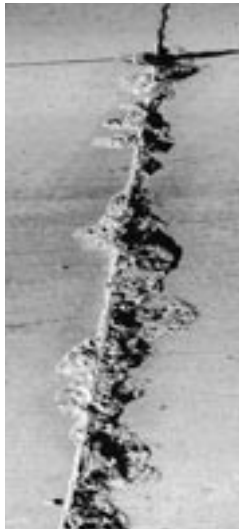
▶▶ Cracks parallel to joint. Dark color next to transverse joint likely indicates D-cracking and additional deterioration. Full depth repair required.
