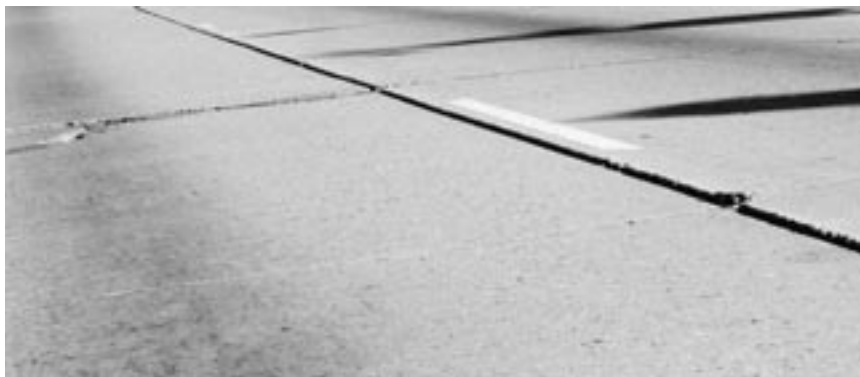
▲ Corner cracking developed into small hole; moderate spalling of transverse crack.
