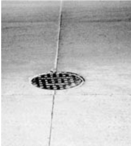
▶ Severe spalling of a transverse joint.
