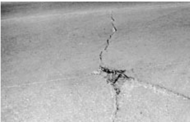
▲ Corner cracking developed into small hole; moderate spalling of transverse crack.
