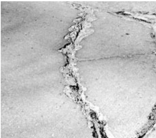
▶ Spalling over shallow reinforcing.
