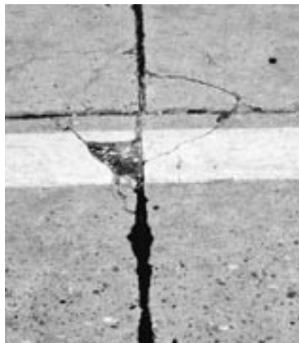
First signs of corner cracking.
