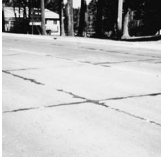
Wide open meander crack (1") with edge spalling. ▼ Corner crack with spalling.
