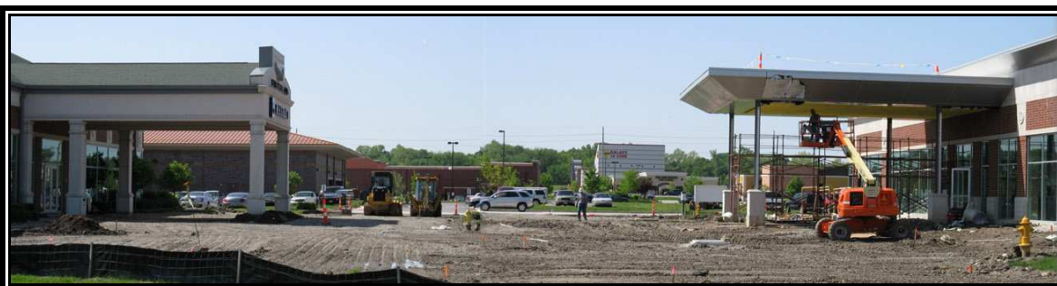
View Looking North at Lots 7 and 8
