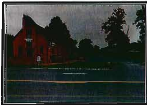
View of Existing Dental Office Building
