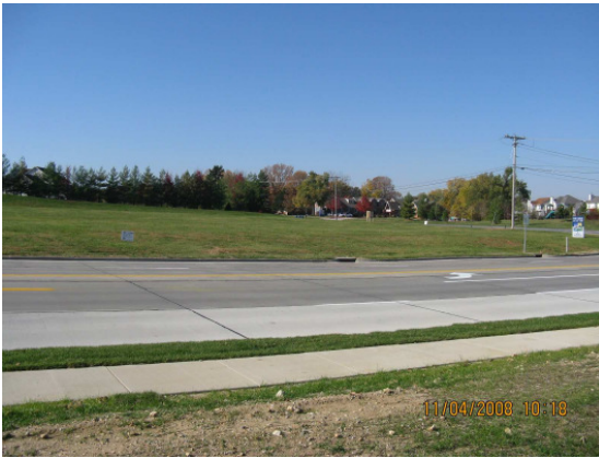
View looking west at C-119 from Baxter Road
