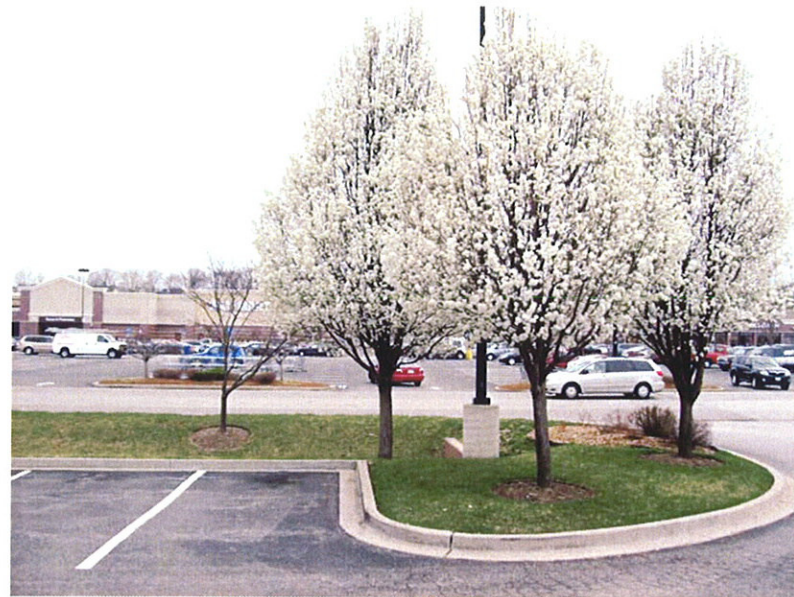
SOUTH SIDE OF BUILDING LOOKING SOUTH
