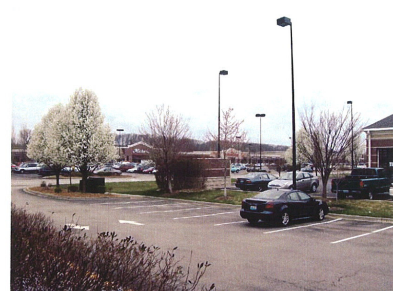
WEST SIDE OF BUILDING LOOKING SOUTHWEST
