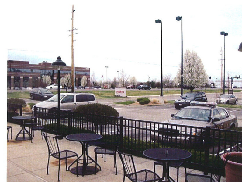
EAST SIDE OF BUILDING LOOKING NE
