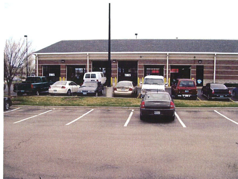
WEST SIDE OF BUILDING LOOKING WEST
