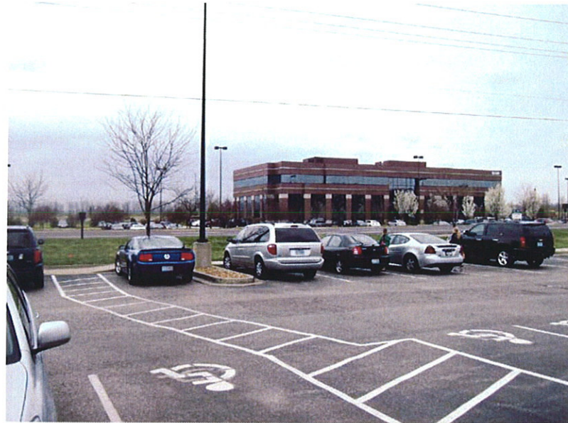
NORTH SIDE OF BUILDING LOOKING NORTHEAST
