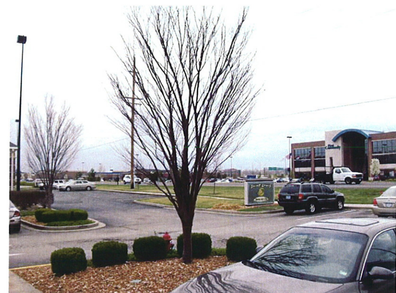
NORTH SIDE OF BUILDING LOOKING NORTHWEST
