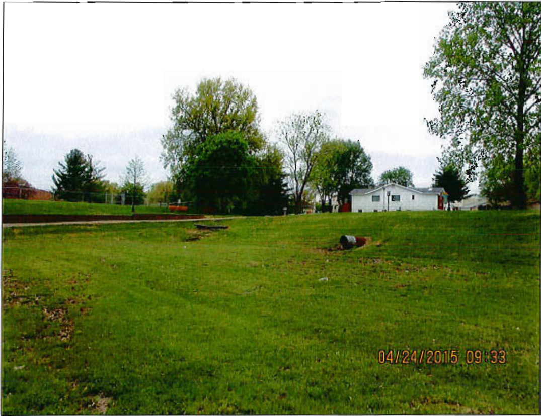
Figure 7: Additional Storm Water Structures
