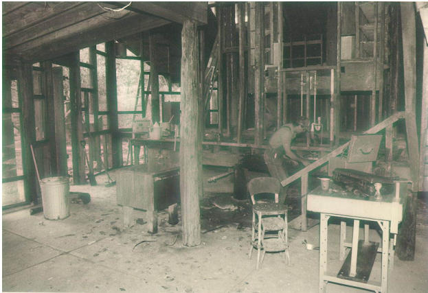
All the walls had to be reconditioned or re-built.
