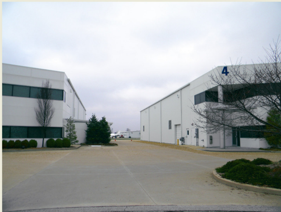
View from N. Bell Ave. looking West
