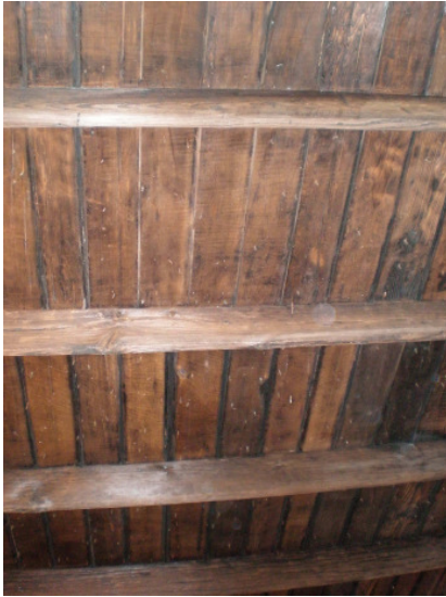
'Aged' rafters in the central hallway.
