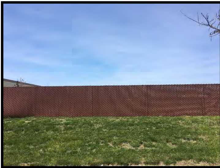
Figure 3: Existing Fencing Material
