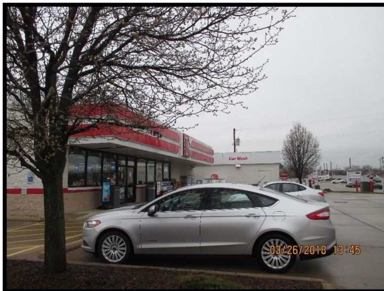
Figure 2: Subject Site from Wildwood Parkway
