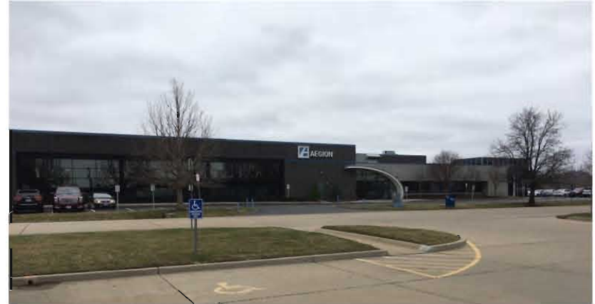
South view: Aegion Headquarters office building
