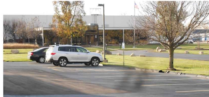
North view: industrial building
