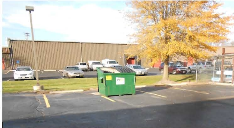
West view: industrial building
