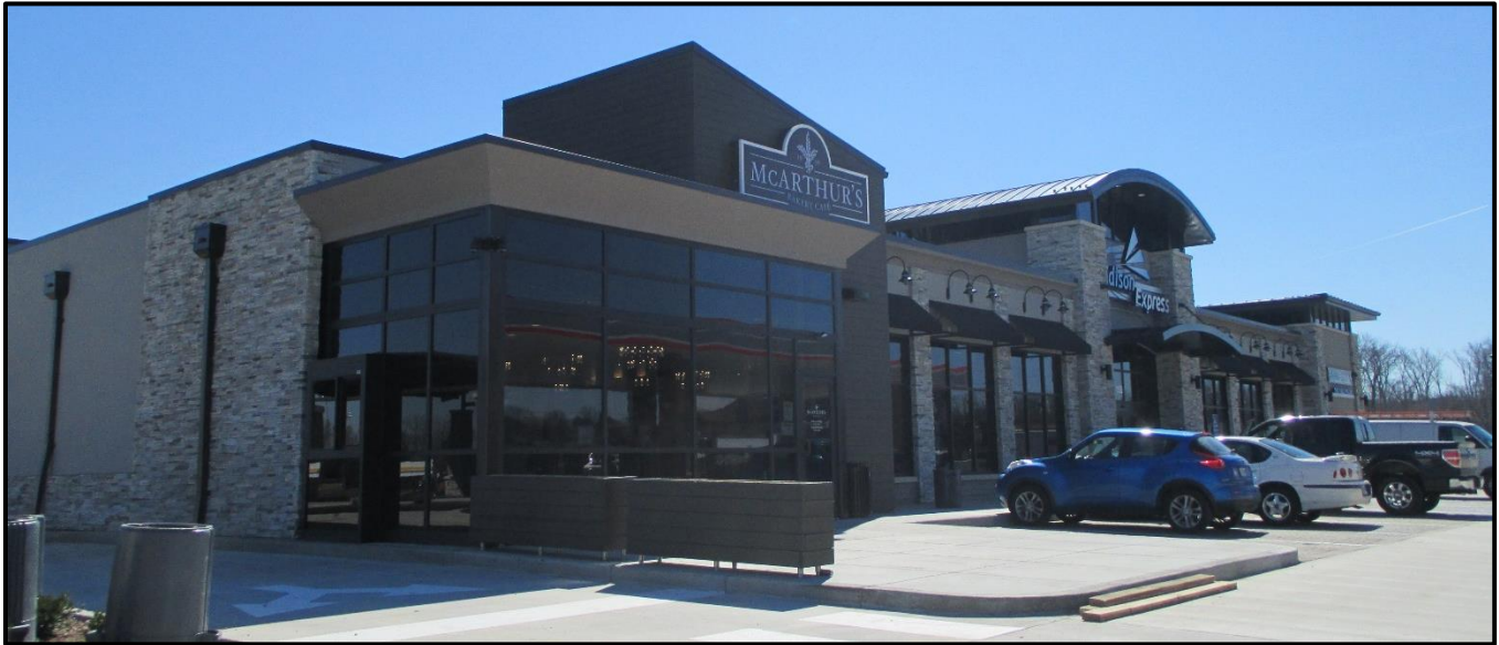
Figure 2: Edison Express wall signage on west elevation (March 2017)
