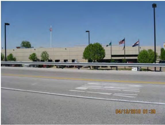
Viewing North at Public Works Office
