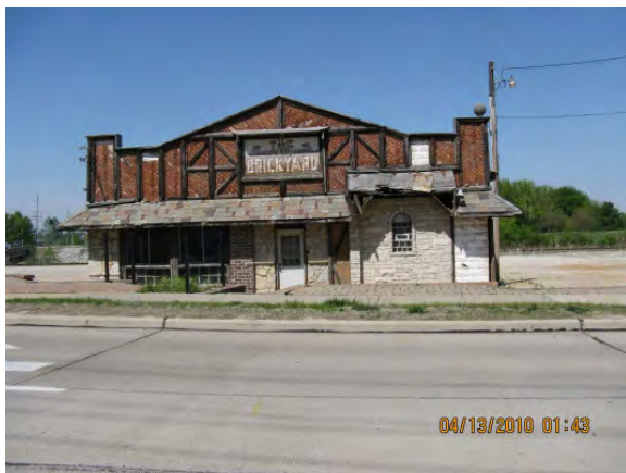
Viewing North at existing structure
