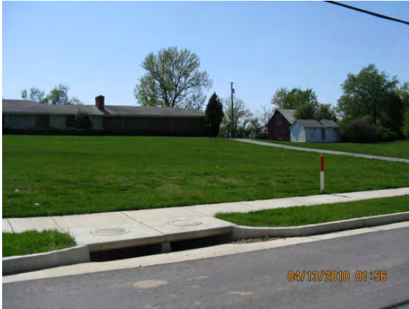
Viewing West at Existing Structures
