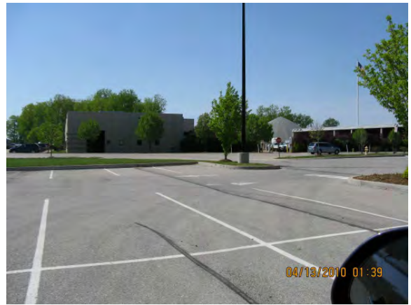
Viewing West at maintenance yard
