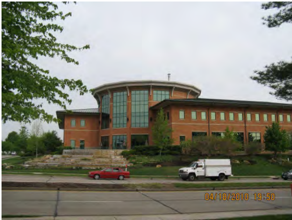
Viewing front of City Hall
