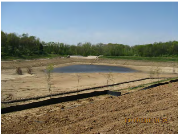
Viewing Northwest at site of Lake 1
