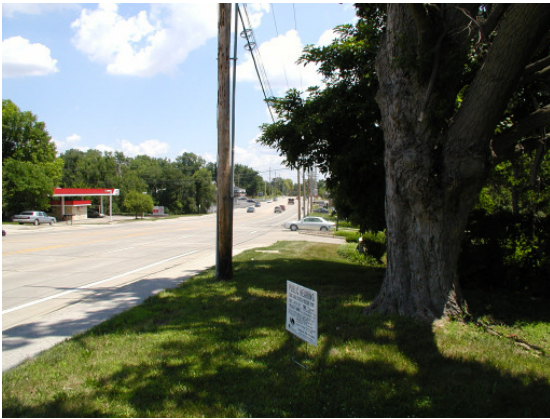
View looking east along Olive.
