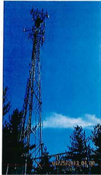
PHOTO OF EXISTING TOWER ELEVATION
