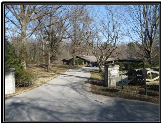
View of the existing residential structure on the property
