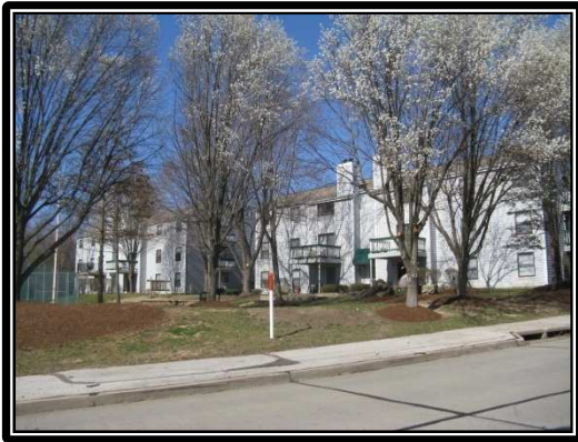
View looking at property east of subject site
