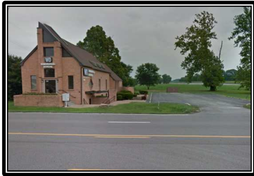
View of Existing Dental Office Building
