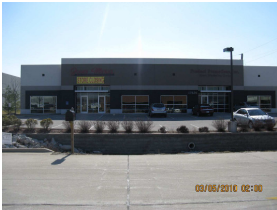
View looking at the site.
