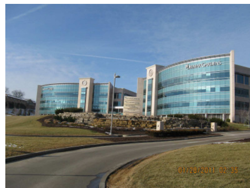
View Looking at existing Delmar Gardens.
