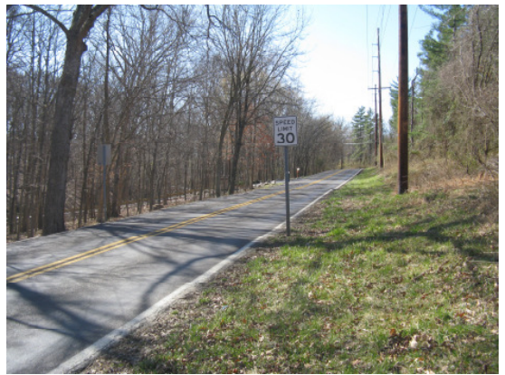
View looking south down Kehrs Mill Road
