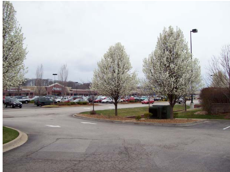
SOUTH SIDE OF BUILDING LOOKING SW
