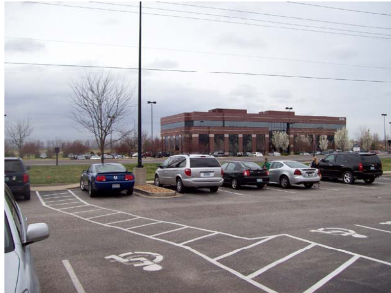
NORTH SIDE OF BUILDING LOOKING NORTHEAST
