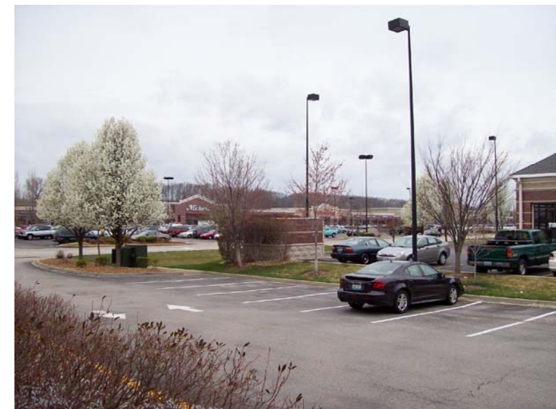
WEST SIDE OF BUILDING LOOKING SOUTHWEST
