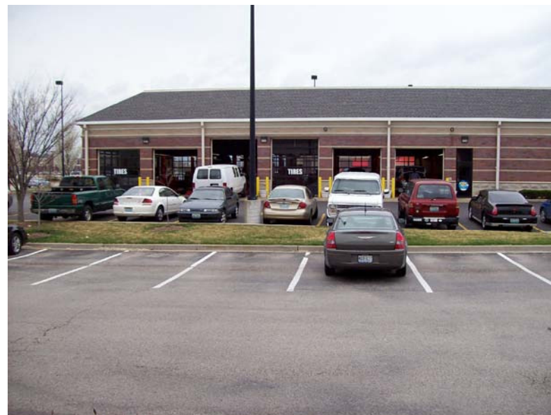
WEST SIDE OF BUILDING LOOKING WEST
