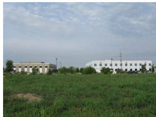
View looking south
