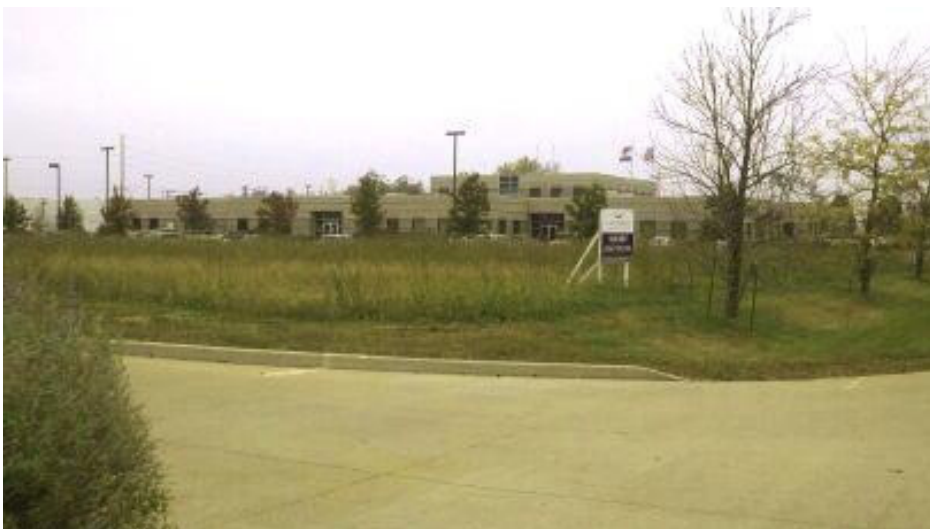
View Looking North West From Entry
