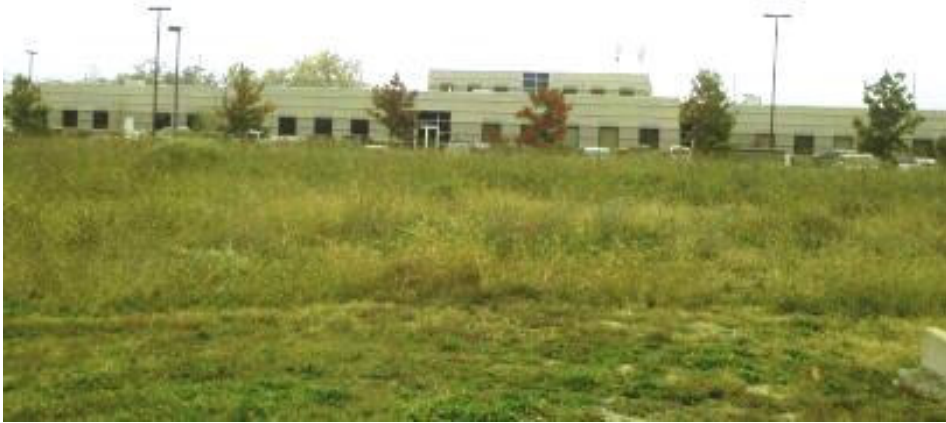
View Looking North From Entry
