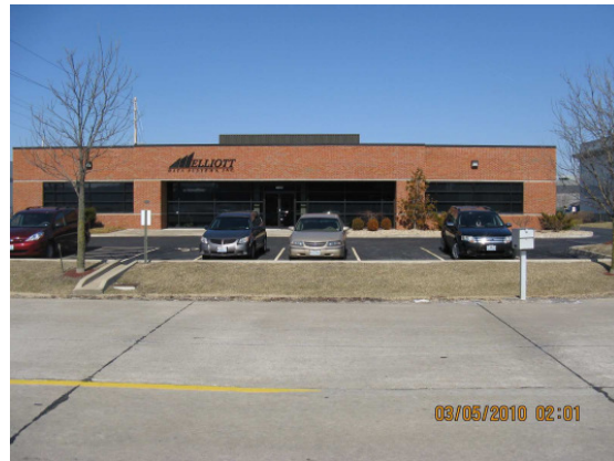
View Looking across Edison Ave.
