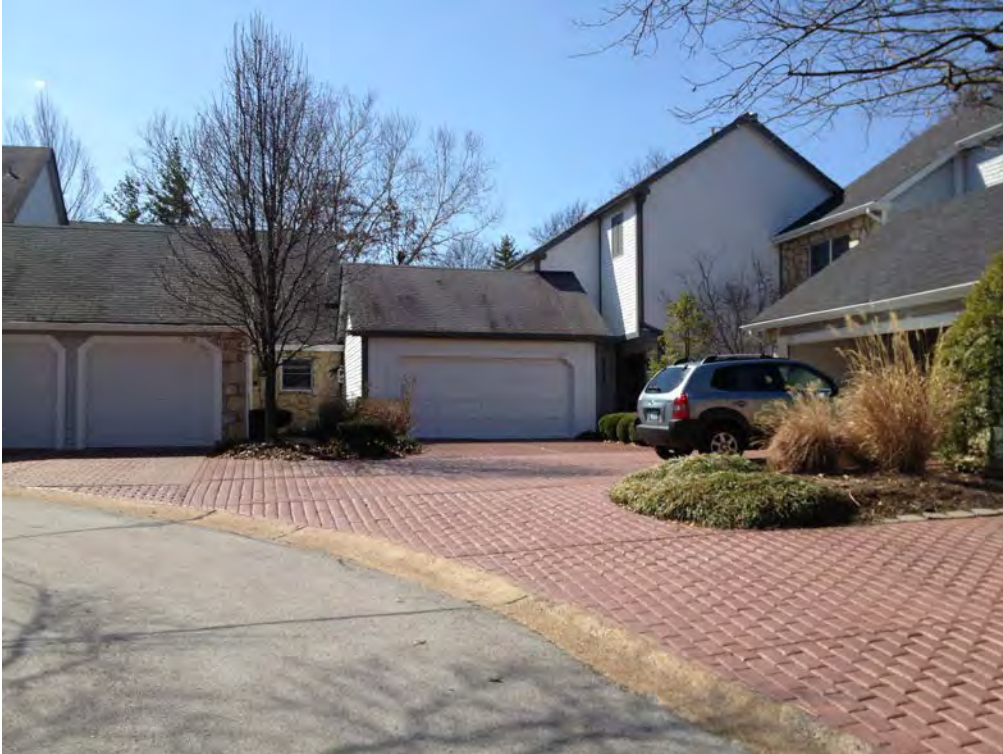
View from looking South directly across from the Eastern edge of the Proposed 4 unit Condo building
