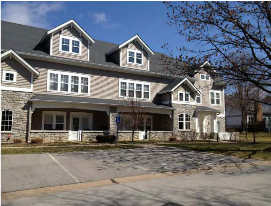
View of the existing building from Milbridge
