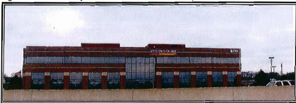
Figure 3: Northern façade of 17107 Chesterfield Airport Road
