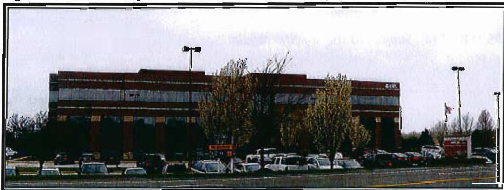
Figure 4: Southern façade of 17107 Chesterfield Airport Road
