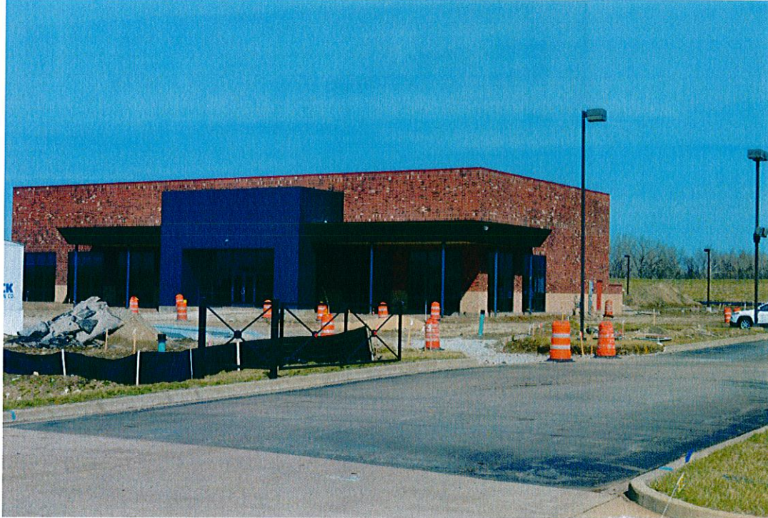
Attempt to stain/paint/change color of entire building (Exhibit G):
