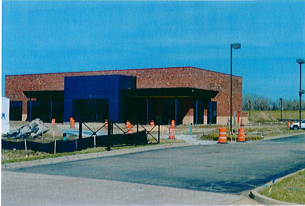
Actual field pictures of new building (Exhibit D):
