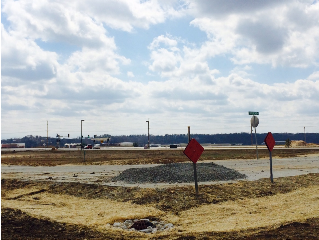
SOUTH SIDE OF SITE LOOKING SOUTH ACROSS CONVENIENCE WAY
