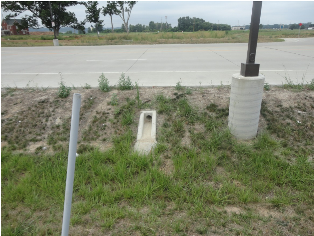
WEST SIDE OF SITE LOOKING WEST ACROSS OUTLET BOULEVARD
