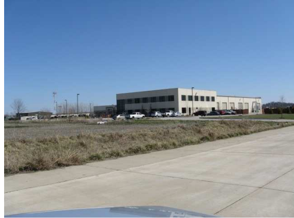
Looking at existing buildings in development.
