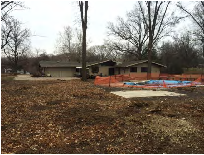
Subject Property Rear View
