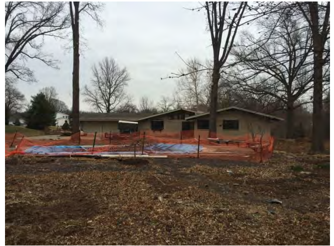
Subject Property Rear View
