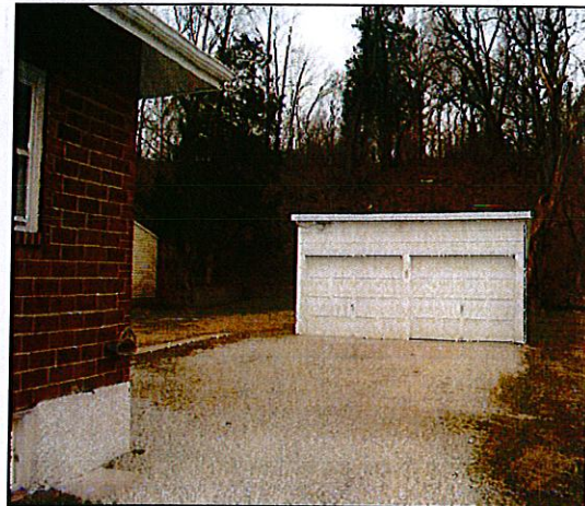
Figure 5: Picture of Garage Interior to Subject Property
