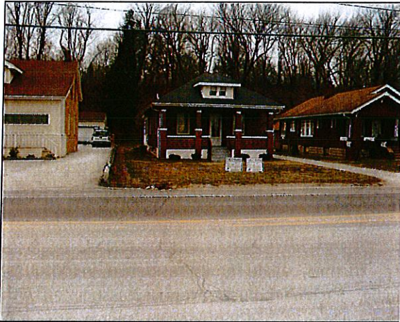
Figure 4: Subject Property from North
