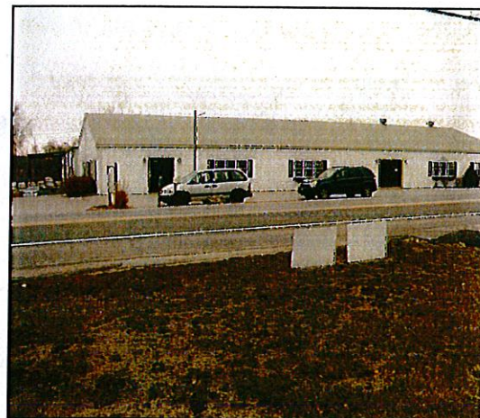
Figure 7: Looking South from Subject Property
