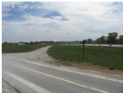
View looking at south end of site from access road and levee trail.
