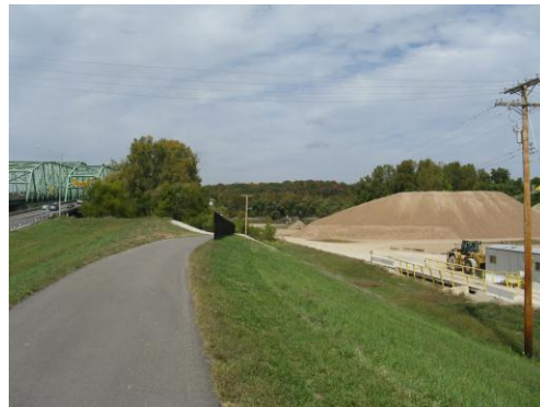
View looking N at Site along Levee Trail.
