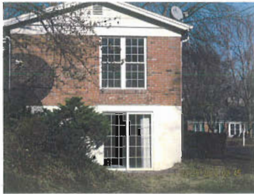
Existing Walkout Basement
