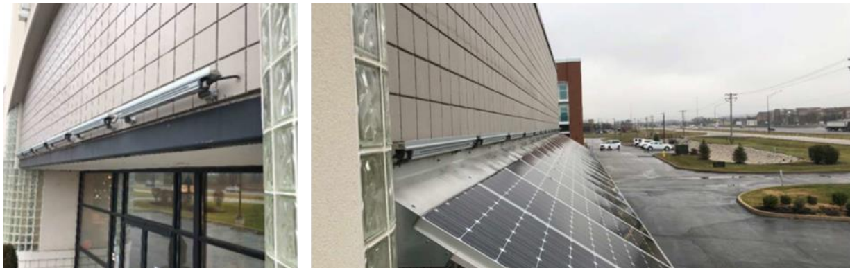
Figure 5: Photos of permanently mounted light fixtures
