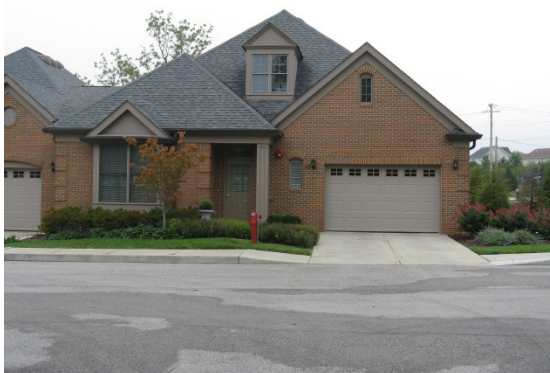
View of one of the Attached Villa units
