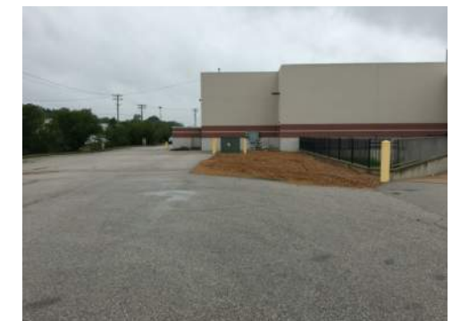
2. EXISTING LOADING DOCK AREA
