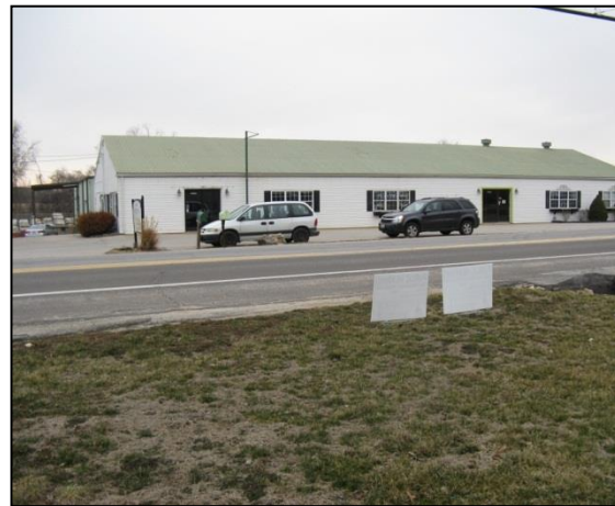
Figure 7: Looking South from Subject Property
