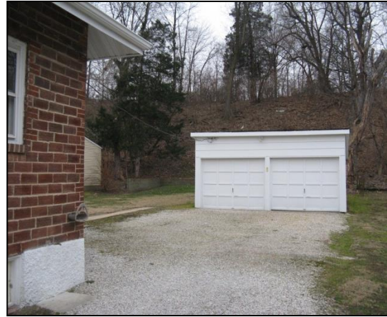
Figure 5: Picture of Garage Interior to Subject Property
