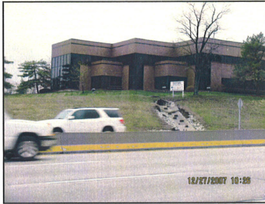
Office building to the south across Highway 64/40.
