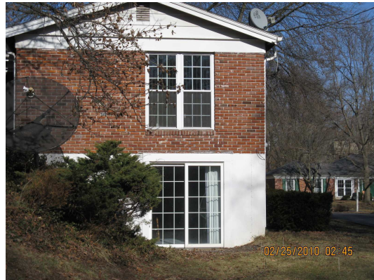
Existing Walkout Basement
