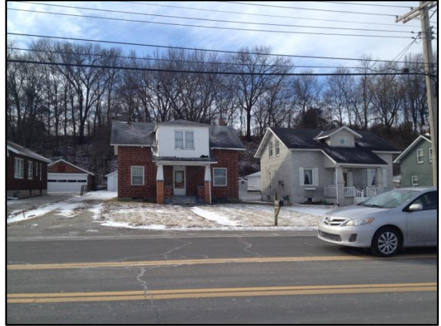
Looking south across Old Chesterfield Road
