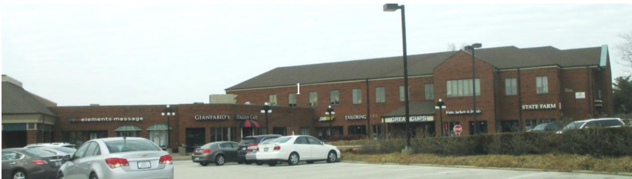
Existing Building D
