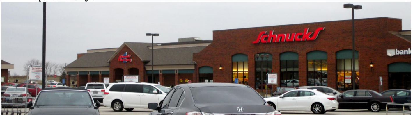
Existing Building C
