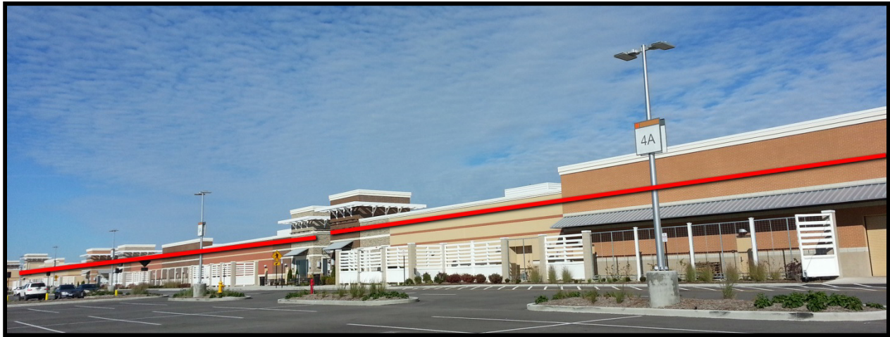
Figure Three: Red line depicts the approximate location of the Existing permitted sign band along the south elevation
