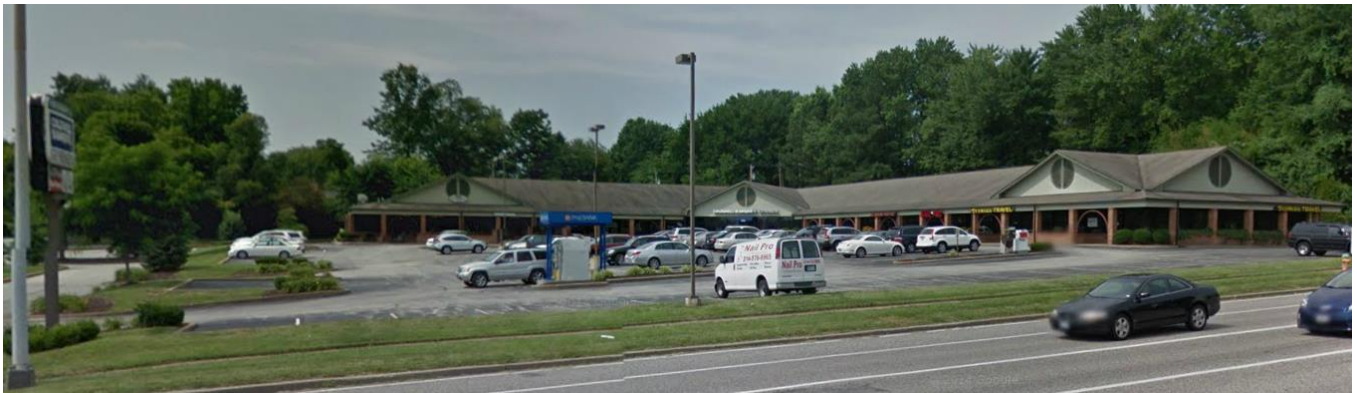
Figure 2 Four Seasons Plaza West Development
