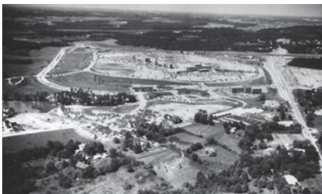
Figure 4— Site of Chesterfield Mall in 1976 (stlcommercemagazine.com)
