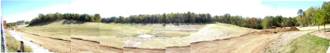
View looking south of the site at the construction of Lake 2
