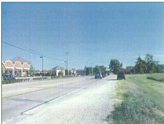
Long Road at Edison Avenue
