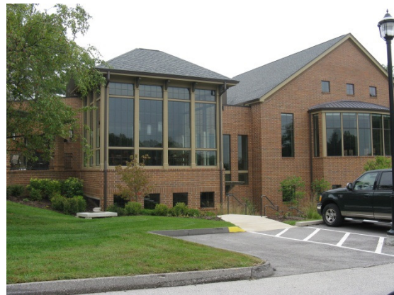
View of the Multi-Purpose addition
