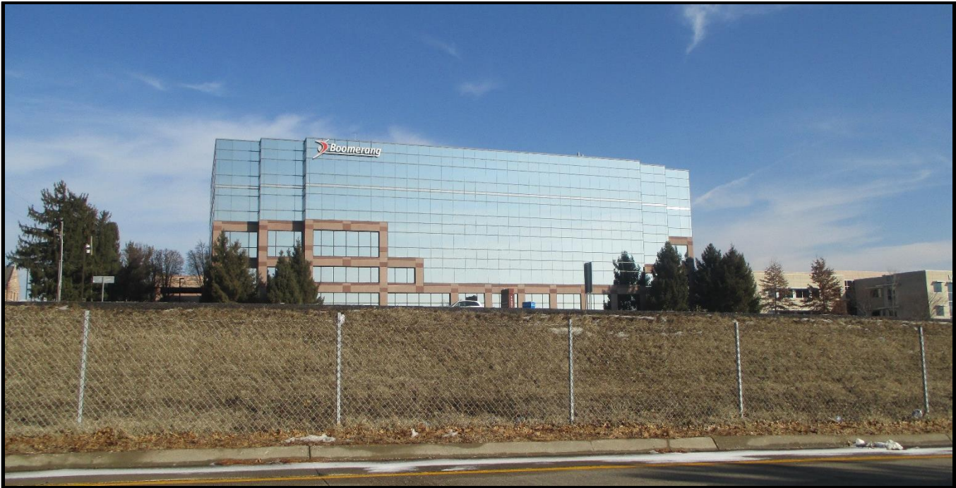
Figure 2: Existing wall signage for the Forty West Office Building (February 2019)
