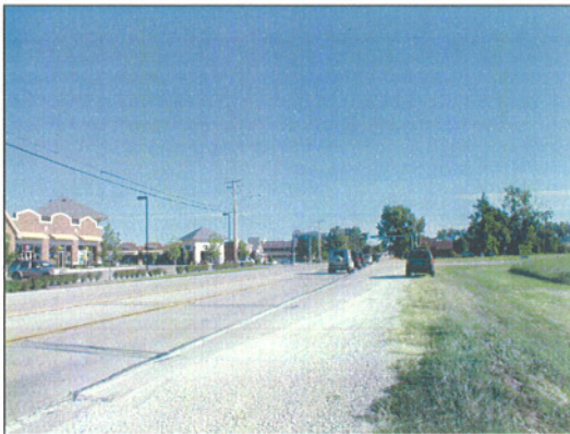
Long Road at Edison Avenue
