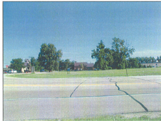
Area north of site-will be Monarch Center
